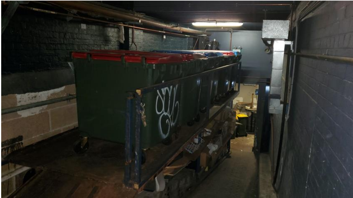
Figure 22: Existing bin storage area facing east
