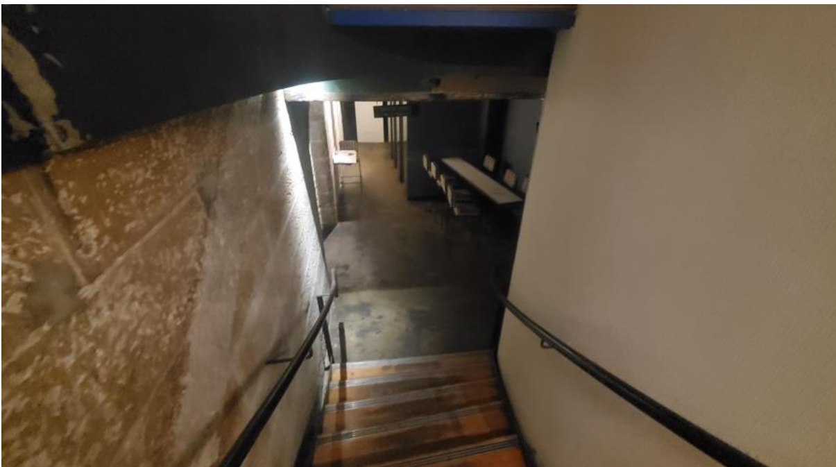
Figure 11: Existing stairs to basement level facing west (proposed to be demolished)
