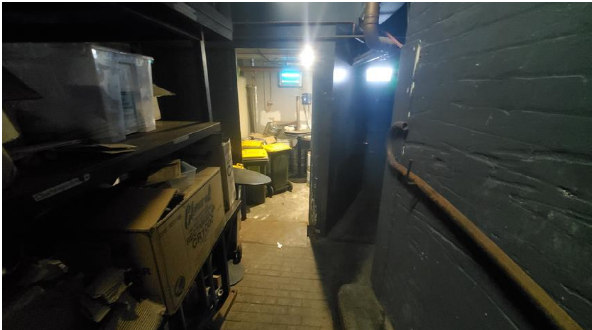
Figure 21: Existing basement level services room facing east
