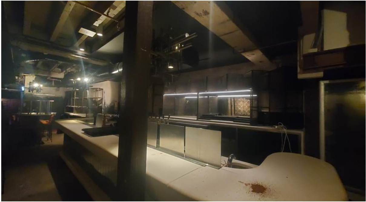
Figure 16: Existing bar area on basement level facing southeast
