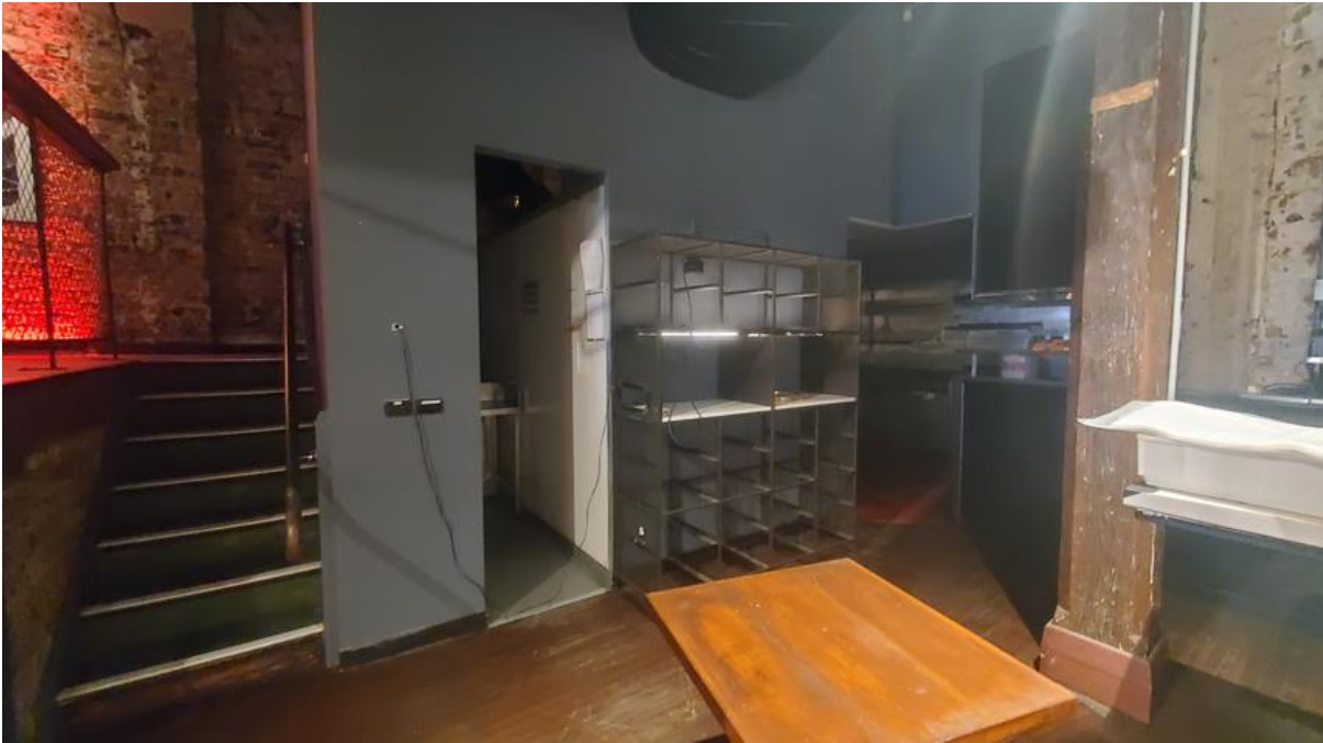
Figure 10: Existing kitchen viewed from ground floor facing northeast
